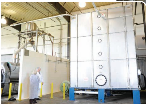
Above, an indoor flour silo with a maximum capacity of 100,000 lb. was recently added to the plant. Right, line operators empty the biscotti dough from a spiral mixer to a trough.
